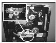
Fig 1: Water Heater Drain Plug
